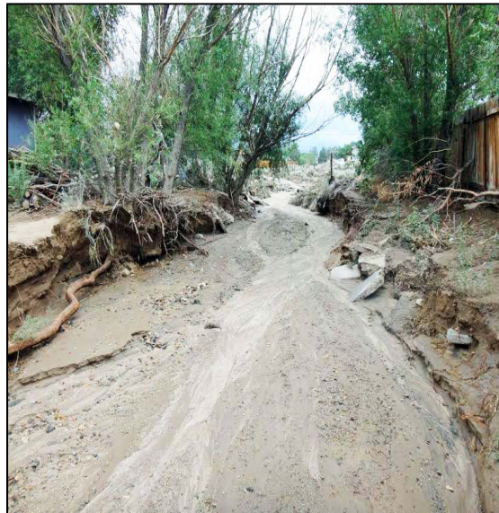
Damage to Johnson Lane drainage ditch Photo credits: John Cobourn/Matt McMackin
