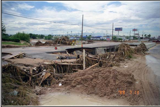
Damage to Boulder Highway
