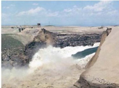
Example of earthen dam collapse: Teton Dam, Idaho, 1976
