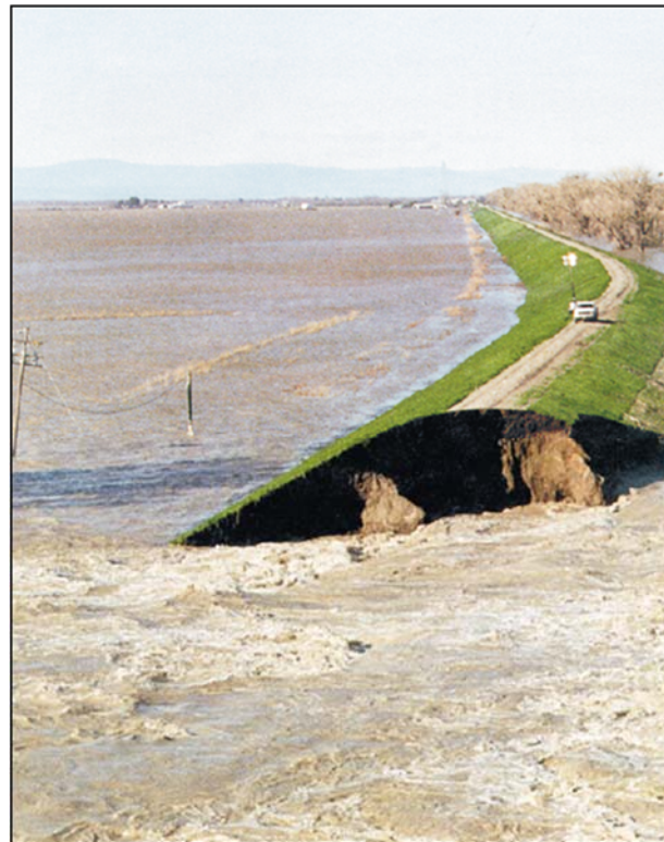
Example of a levee breach
