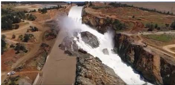
Example of damaged spillway: Oroville Dam, northern California, 2017
